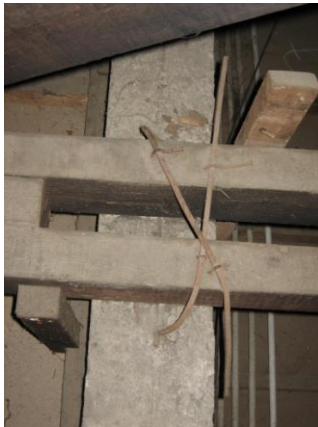
Improper fixation of roof girder, Indonesia GI
