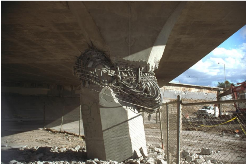
Collapse, elephant footing, influence of horizontal and vertical acceleration
