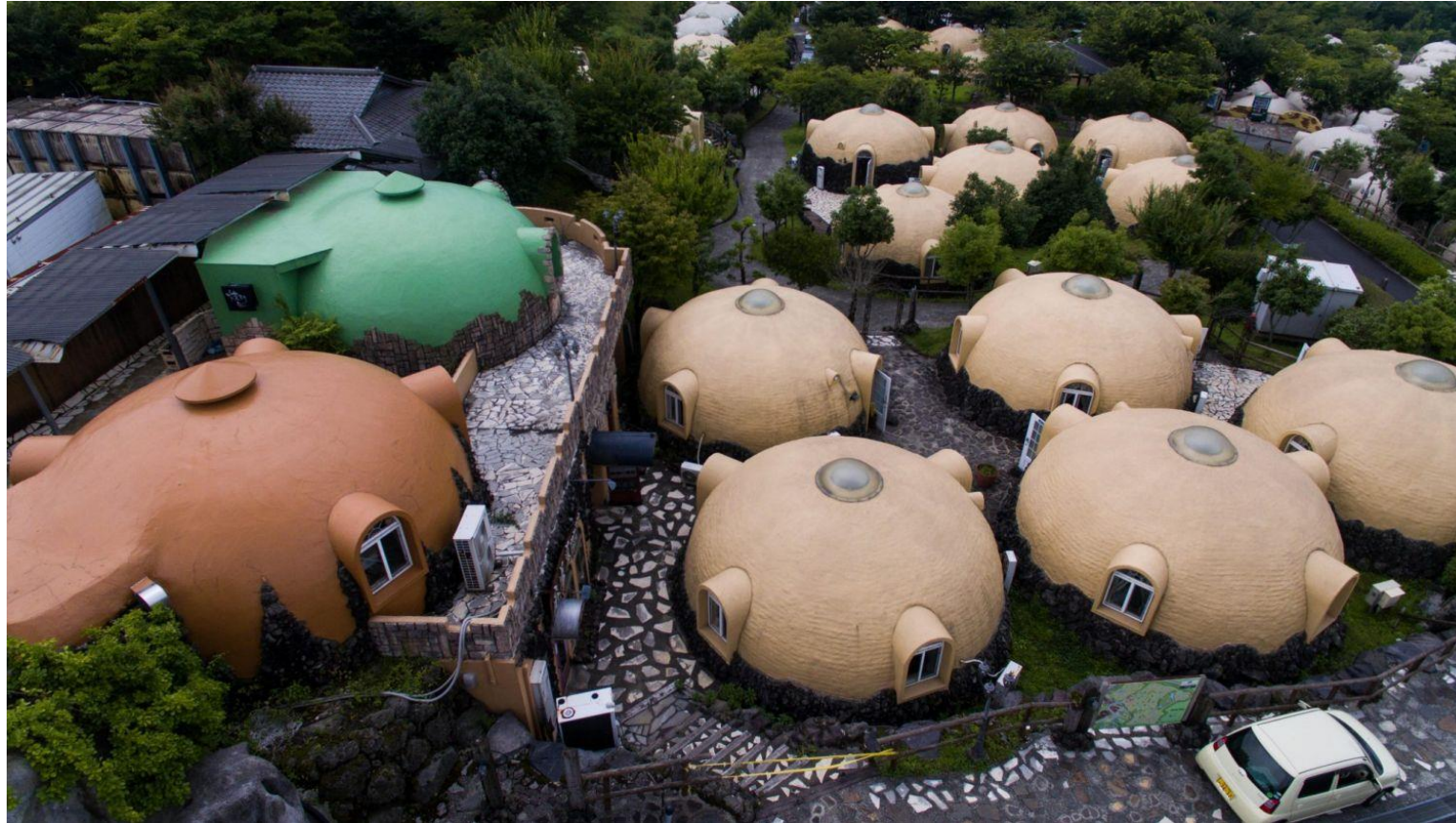
Aerial view of earthquake-resistant dome houses in Aso Farm Land, Kumamoto prefecture, Japan, made of styrofoam. Photo: Alamy. (Wikipedia)
